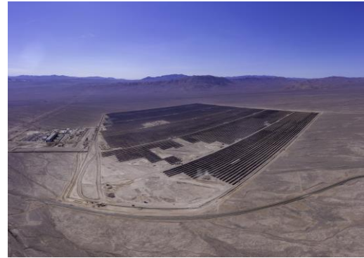
68MW / 418 MWh BESS Tamaya (storage) US$128 million investment
