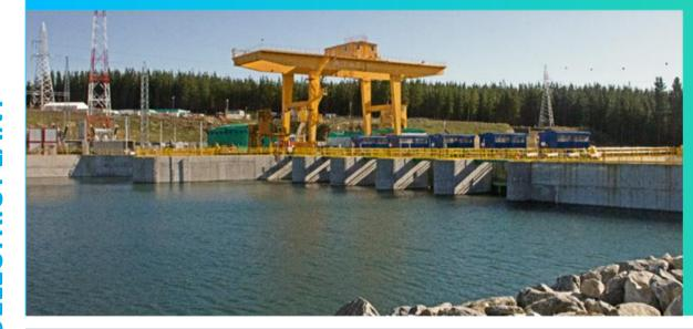
34MW run-of-river, 14Mm3 reservoir ~60km of Los Angeles, Bío-Bío. Operating since 2015. Powerhouse w/2 17.2MW Bulb-Kaplan units
