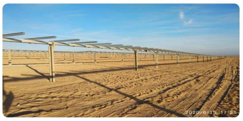
15.6k drill holes, 13k steel piles, 205 trackers, 11k solar modules assembled
